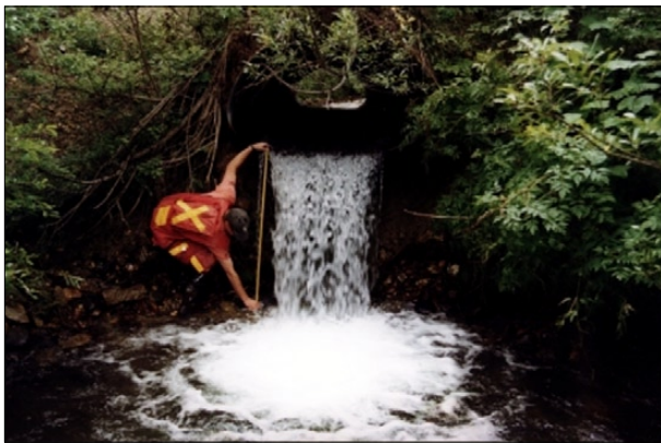
FIGURE 2. Culvert going under the lower Torpy road at stream 19 (July 1999).
