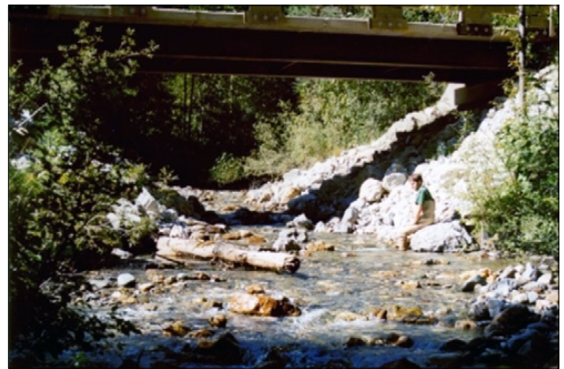
FIGURE 3. Bridge on the lower Torpy road crossing stream 26 (July 2000).
