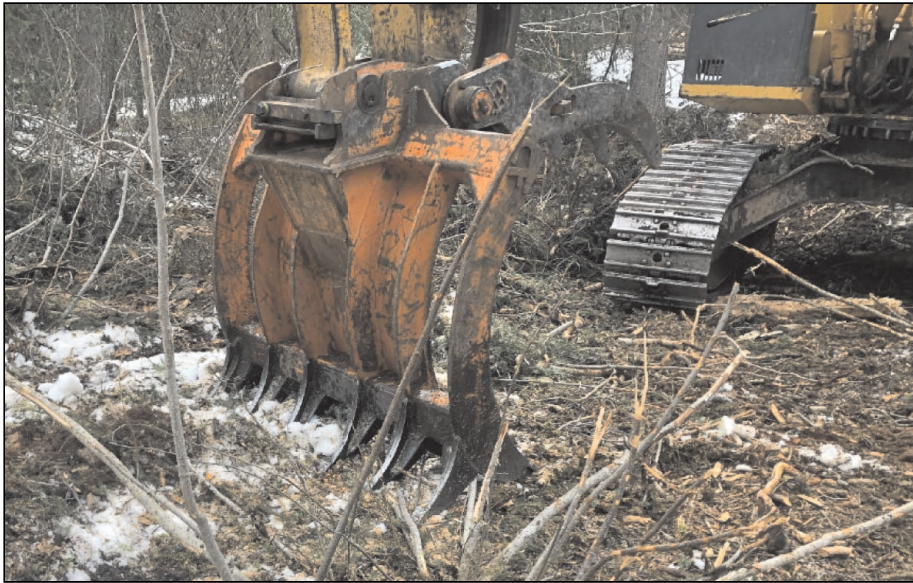
Figure 3. Image of excavator with modified brush-rake attachment used to collect fine fuels in the Burns Lake Community Forest in mechanically raked fuel treated units.
