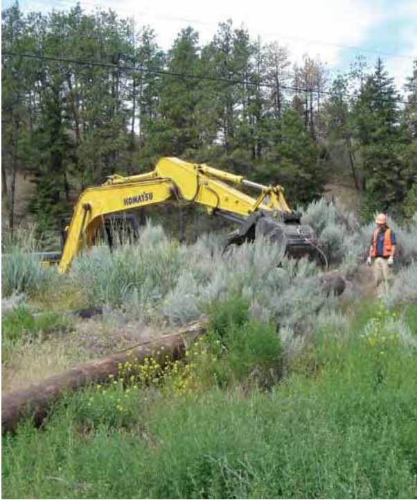
FIGURE 2. Using heavy equipment to deactivate old roads.
